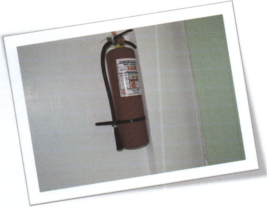
Near EXIT door
