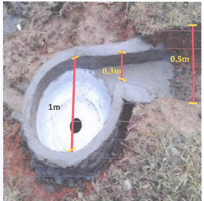
Figure 12. Design of the Cylindrical Concave Basin
