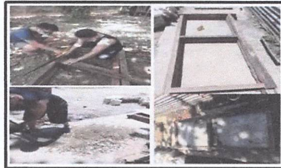
Figure 6. Preparation and making concrete slab
