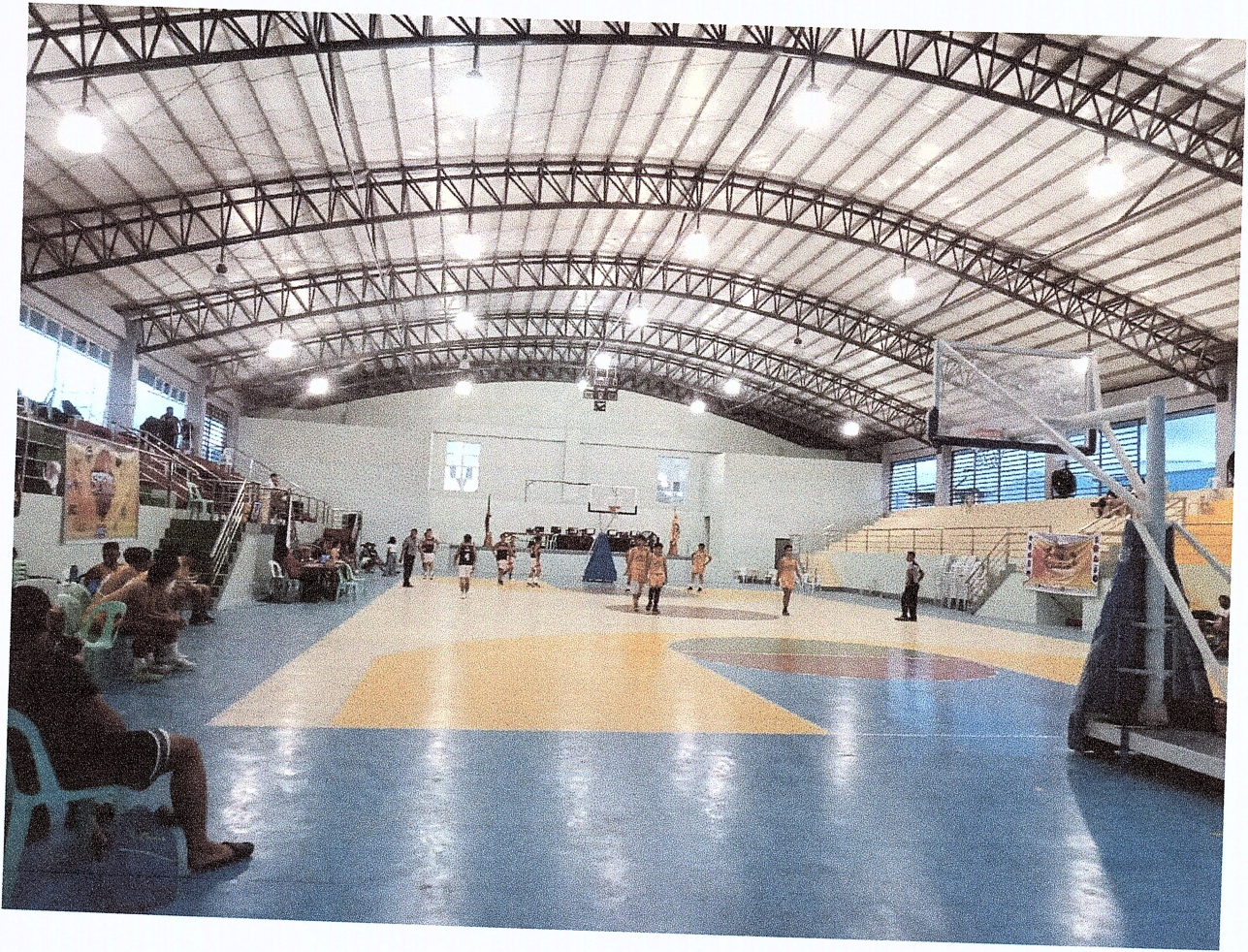
Lighting and Ventilation
