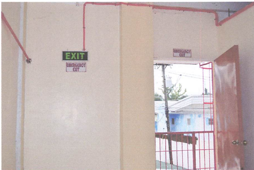
I.6 Floor plans indicating fire exits and location of fire-fighting equipment, stand pipes, and other water sources are conspicuously displayed in each building.
